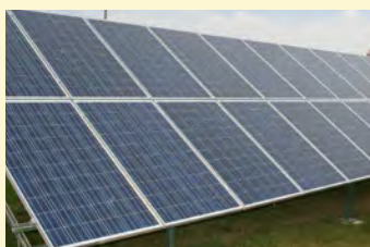
Multicrystalline or polycrystalline solar cells
