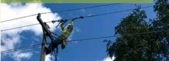
**STORMS:** Following a late-August storm, a tree fell into ECI REC's distribution line east of Rowley, causing it to burn down. Crews were dispatched. Because the line fell in a private right of way, Lineworker Grover had to climb the pole to put the line back up.
