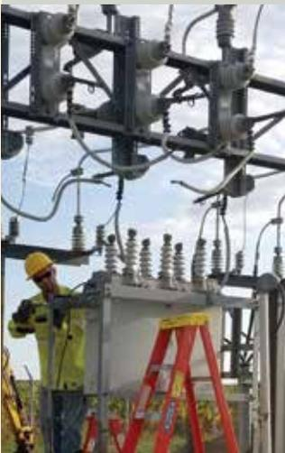
**SUBSTATIONS:** Lineworker Donnelly conducted regular maintenance at the Sumner substation. He changed out the oil circuit recloser and updated the wire size for the substation's upcoming capacity upgrade.
